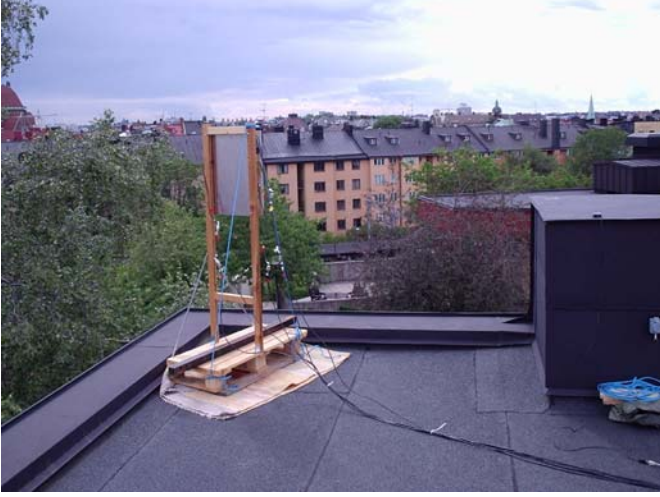
Figure 1: View of “Kårhuset-A” Base-Station.
