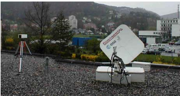
Figure 6. A fixed Satellite Earth Station and a FSO system at the top of the building of the staff department MilDiv ST
