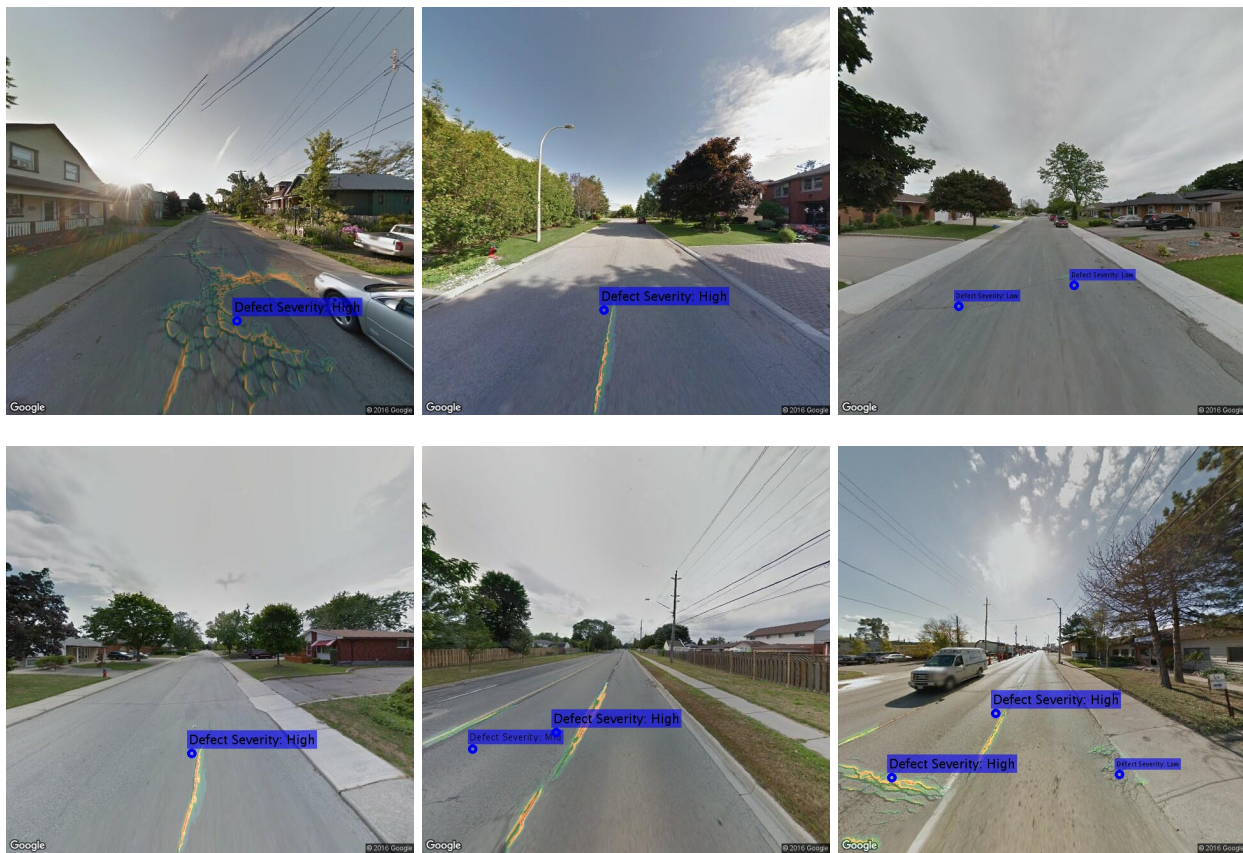
Fig. 4: Sample crack detection results of our algorithm. The crack detection scheme displays per-pixel severities of detected defects in blue and green for ‘mild’ defects, orange for ‘medium’ defects and red for ‘severe’ defects. The blue boxes contain information about the severity of the defect instance as a whole, using information collected from the per-pixel severities.
