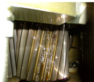
Fig. 7. Broken Pinion on Intermediate Shaft
